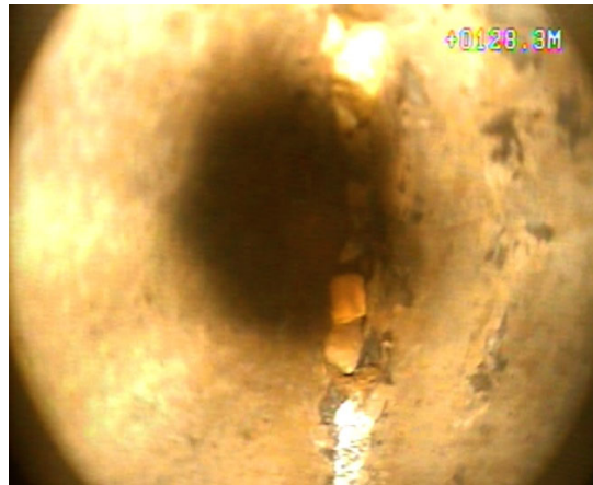
Slotted aperture at 128.30m noted to be heavily corroded with gravel ingress into bore occurring.
