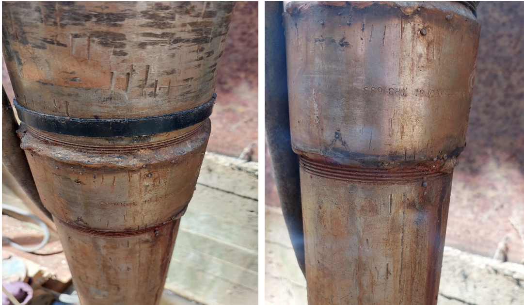
Condition of pumping equipment showing welded couplings.
